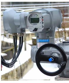
At Marienheide WWTP. around 20 AUMA actuators with Profinet interface are linked in a ring topology with built-in redundancy.
