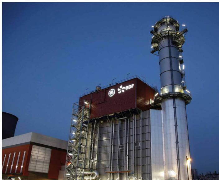
With a record thermal efficiency of 62.22 percent Bouchain combined-cycle power plant (CCPP) was rated the world's most efficient gas-fired power plant by Guinness World Records. The plant uses a single GE 9HA gas turbine and has a generating capacity of 605 MW. To achieve such high efficiency, GE deployed an advanced distributed control system based on Foundation Fieldbus (FF) communication. For this reason, actuation technology supporting Foundation Fieldbus was required.
